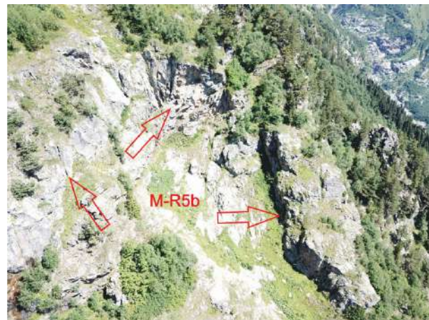
Fig. 4-9: Release area M-R5b. View to the northeast.
