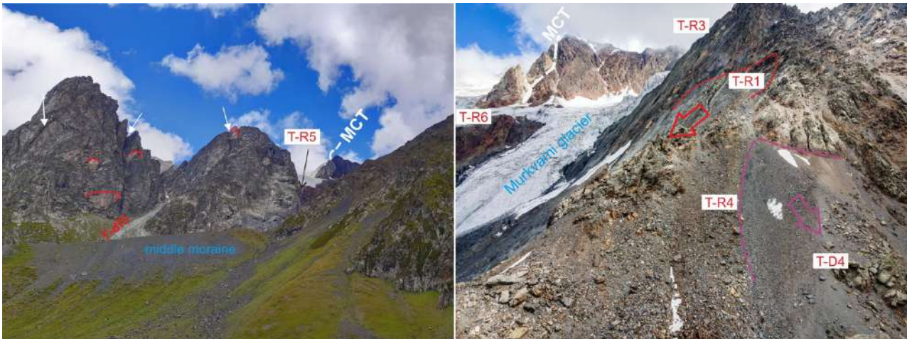
Fig. 3-6: Left: Northward view to crystalline rock towers of Main Range Zone at the northern margin of the tributary with multiple minor rockfall detachments and active cracks along which medium or large volumes might detach in the future (see also Attachment 1). Right: Detachment areas T-R1, T-R3, T-R4 and T-R6 and deposition area T-D4. View to the northeast.
