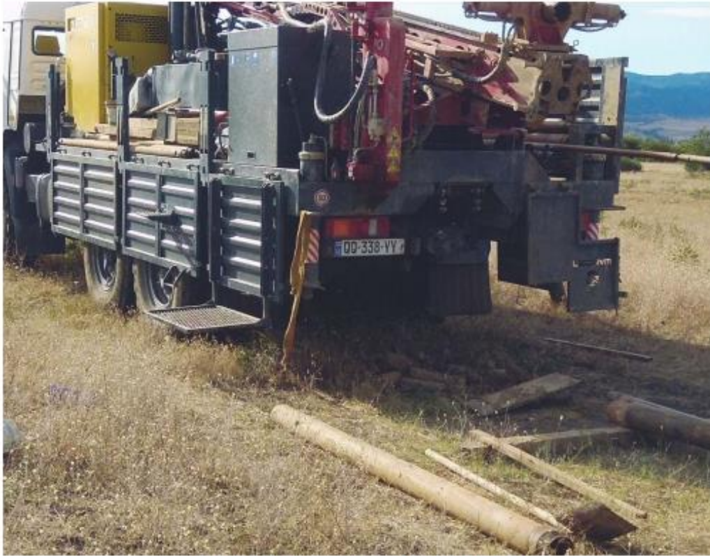
Photo BH1-1. Location of Borehole BH1
