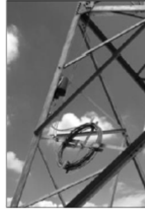
Installation on tower
