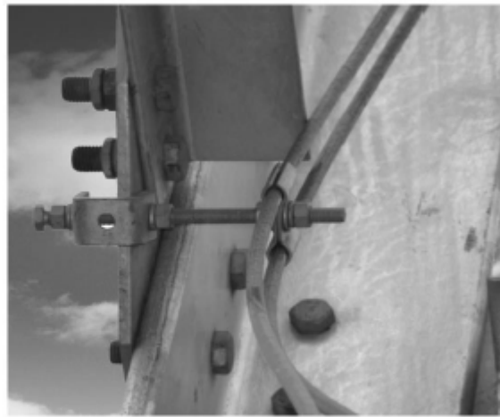
Installation on tower
